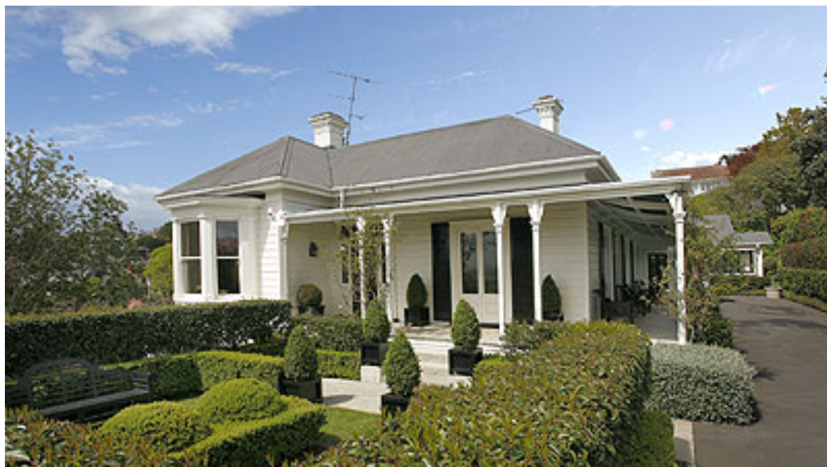
Figure 1: North and partial west elevations of 35 Seaview Road (L. Esler collection).
