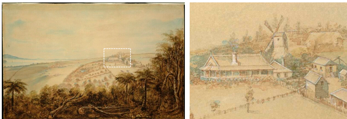
Figure 3: (Left) A painting (attributed to Henry James Warre) showing a view of Parnell from the Parnell entrance to the Auckland Domain, c.1850s. Major Matson's residence 'Brookside' stands on the corner of Birdwood Crescent and Parnell Road. (Right) A close-up of 'Brookside' (B-061-006, Alexander Turnbull Library, Wellington).
