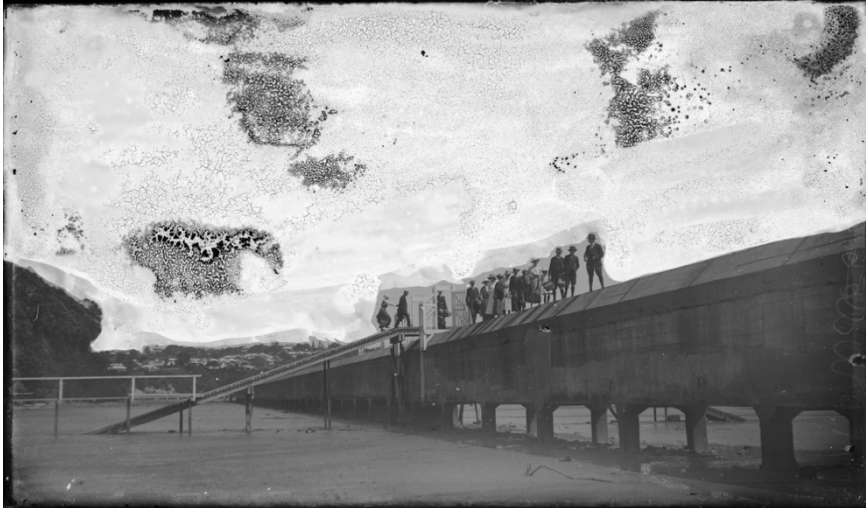
Figure 4: Photograph showing a group of people standing on top of the Hobson Bay sewer, date unknown. Note that the jetty has been constructed, which extends up and over the sewer (Auckland Libraries Heritage Collections, AHJ-G-191).
