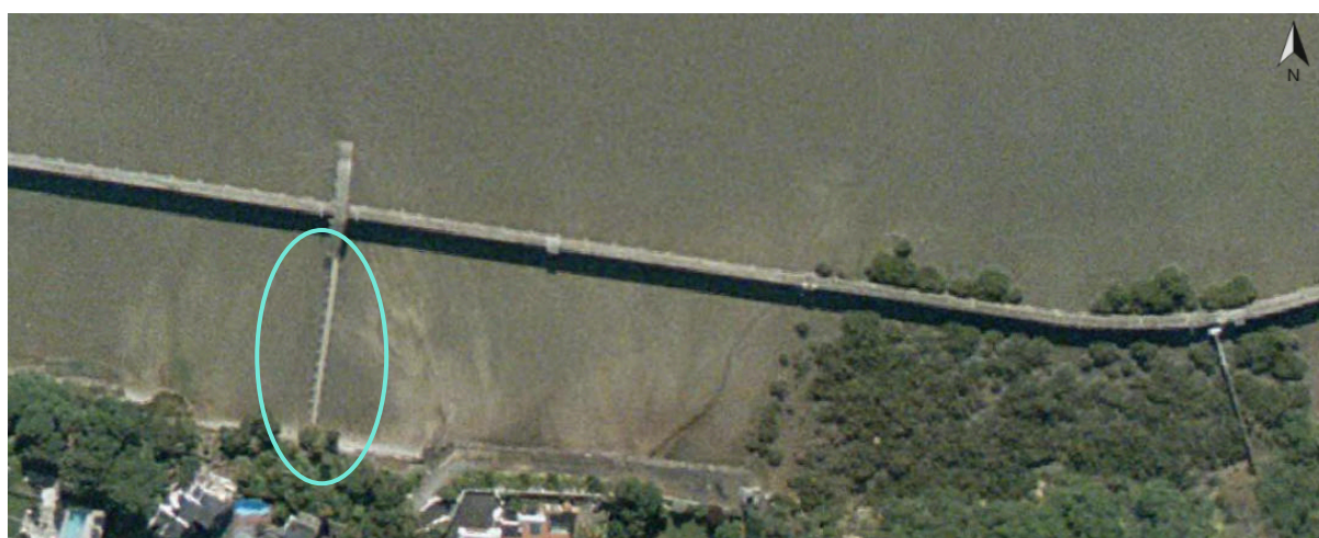
Figure 10: Series of aerial images (from top to bottom) 1940, 1959 and 2008 showing the Wilson's Beach Jetty (circled). Note in each of the images the jetty extends out into the bay and extends up and over the main sewer line (Auckland Council Geomaps).
